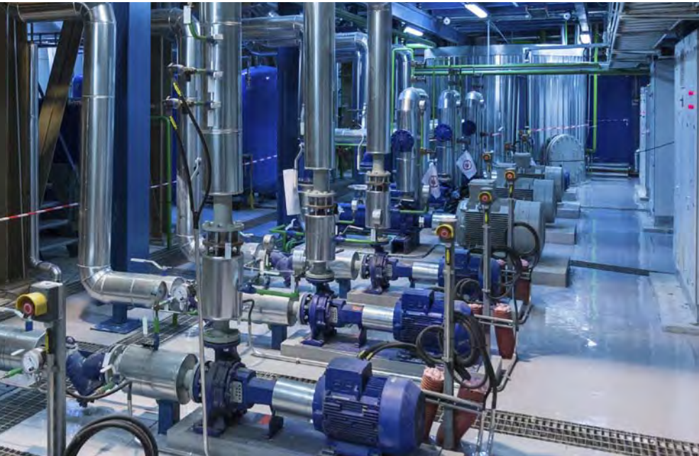
Pump applications, e.g. for building automation operate energy-saving with frequency inverters
